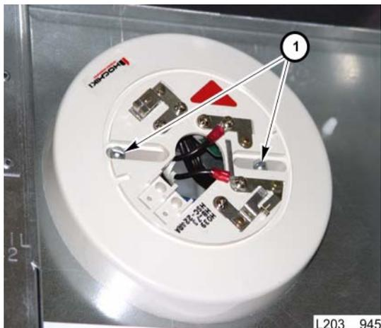
1. Position the replacement base assembly on the mounting plate and secure with two screws (1).
