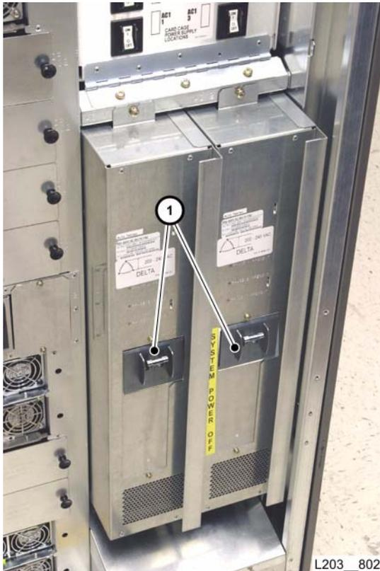
3. Set PDU circuit breaker(s) (1) to OFF (down).
