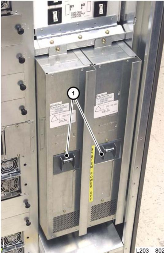
8. Set PDU circuit breaker(s) (1) to ON (up).
